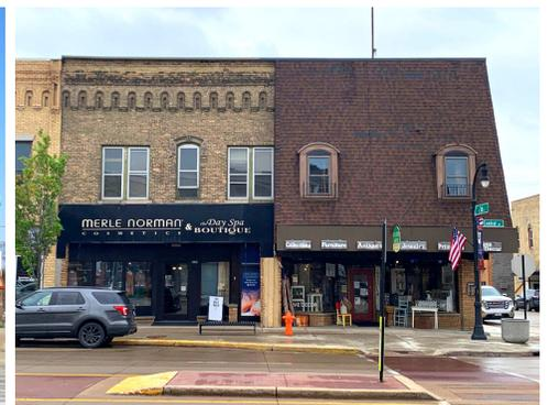
If a rigid canopy is preferred over a canvas awning, it should only span the window or door opening, not the entire façade. Right: A poor example of rigid canopy. Far right: A better example of rigid canopy.
